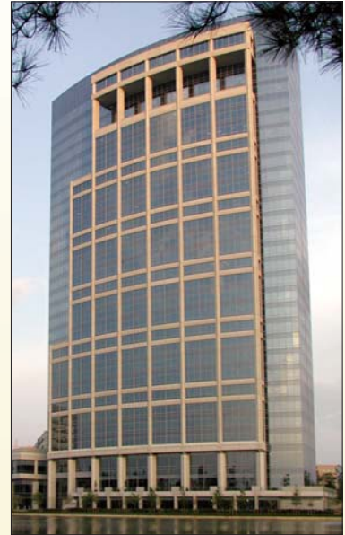
OneSource's work at this Petroleum company's headquarters included scalable software for access control, including more than 400 prox readers.
