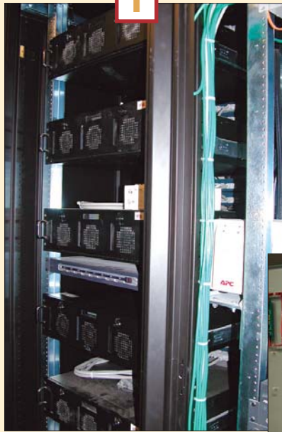
1. The CAPA installation includes nine rack-mounted Lenel DVRs. Each one is capable of accepting 32 cameras.
