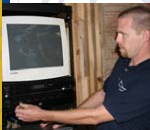
Technician Lee Rowland adjusts a rack containing audio/video components such as DVR, audio receivers, CD players and cable boxes. The setup provides adequate
