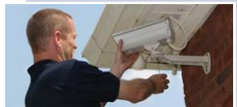
Life & Property Security Systems Technician Lee Rowland carefully calibrates one of four cameras connected to the home’s CCTV system. This camera is larger because it is used to keep an eye on the marina area some 400 yards away.
